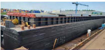
An old lady passed its inspection for certificate renewal
